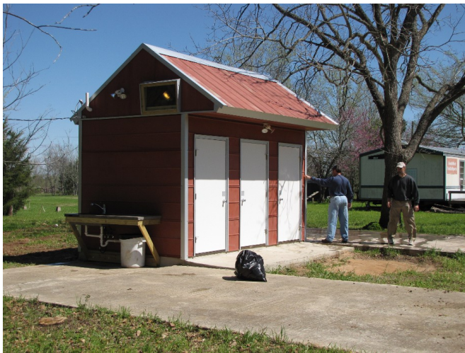
The new bathhouse at Hidalgo
